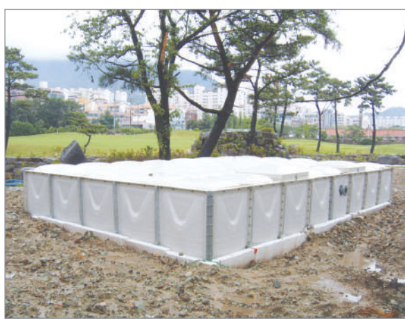
Reclaiming Type Tank
